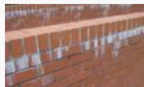
Lime stains emanating from mortar. No damp proof membrane has been incorporated under the brick edge capping.
